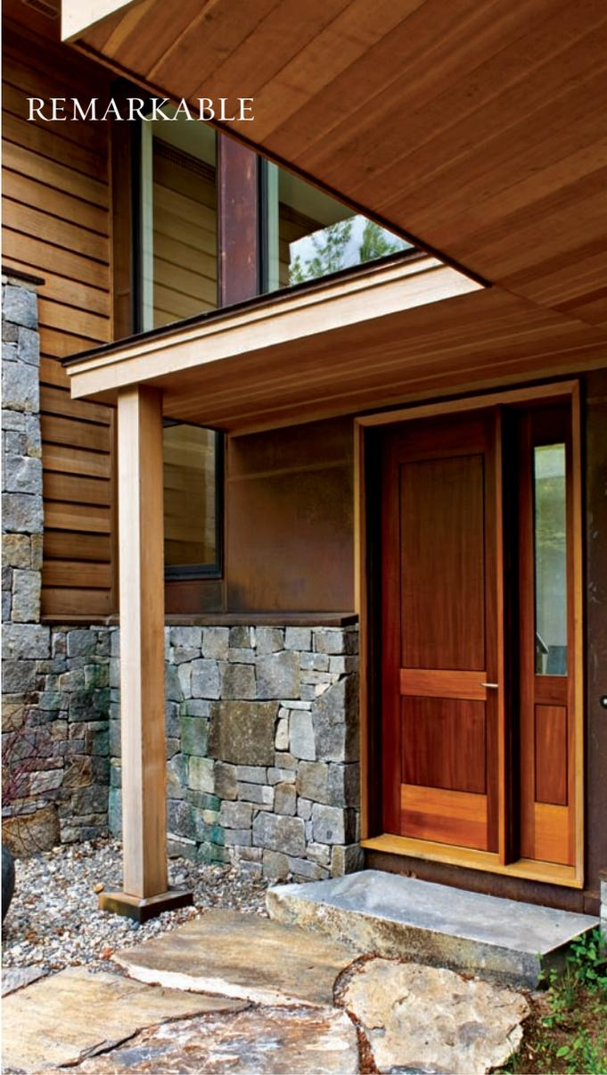
Vertical-grain Douglas fir was used for the soffit (above) and for the ceiling in the enclosed porch. The bold eaves not only help protect the house from the elements, but they also add to the natural shade provided by the neighboring trees. “The owner was drawn to the site and to the Prairie Style roof for a very practical reason,” Van Dam says, “he didn’t want too much sunlight.”
